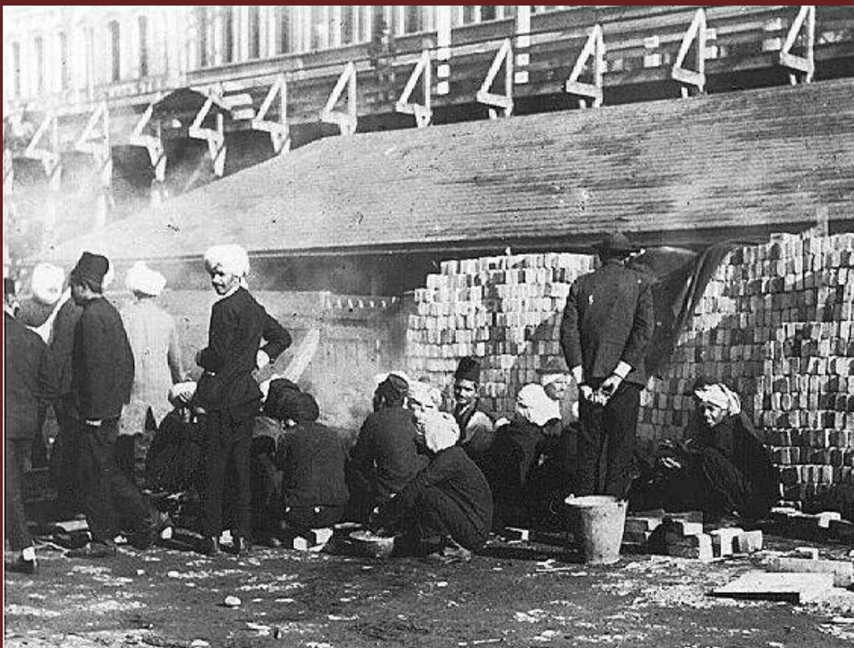
Sikh brick workers in British Columbia
